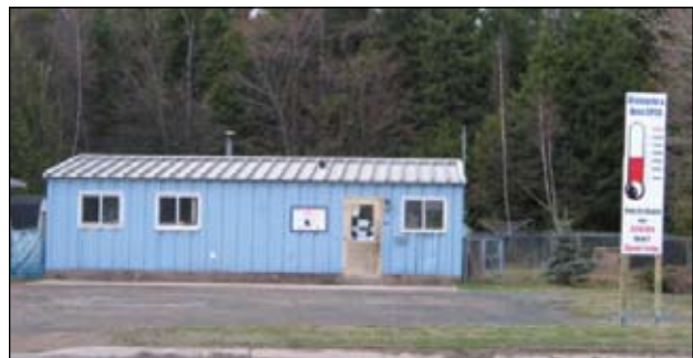
The 35 year old facility in desperate need of repair. Photo: Oromocto and Area SPCA
